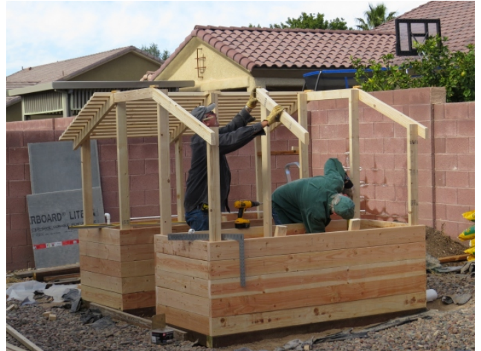
Elevated planters in progress à la the Lynn Brothers
